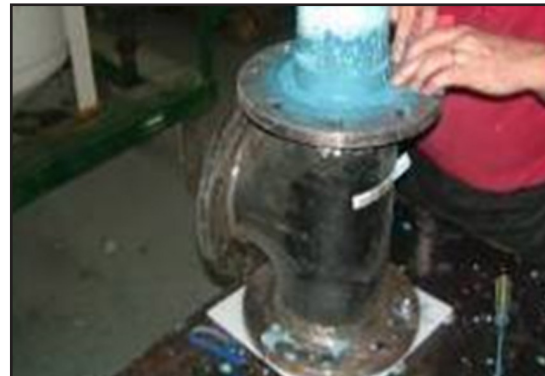
Compacting ARC MX1
